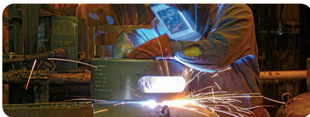
The engineering unit workshop fabricates and mills industrial machinery and equipment as per design specifications
