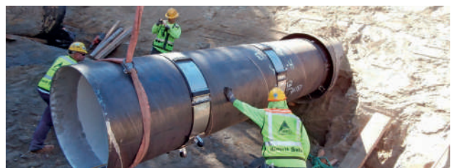
Steel line pipes are used in transmission pipelines in the oil and gas, and water and sewage sectors. The line pipes are also used as piles at ports and jetties
