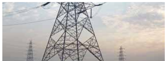
Secure reliable power sourced from CS Energy
