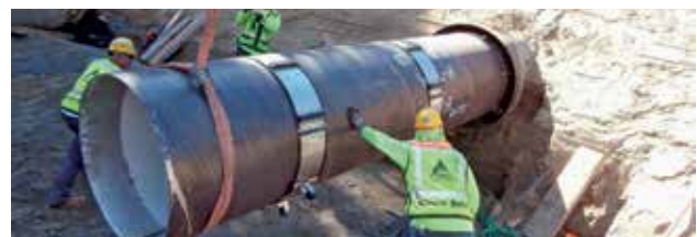
Steel line pipes are used in transmission pipelines in the oil and gas, and water and sewage sectors. The line pipes are also used as piles at ports and jetties
