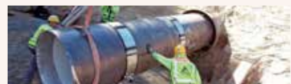
Steel line pipes are used in transmission pipelines in the oil and gas, and water and sewage sectors. The line pipes are also used as piles at ports and jetties
