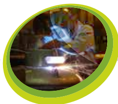
The engineering unit workshop fabricates and mills industrial machinery and equipment as per design specifications
