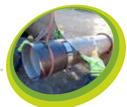
Steel line pipes are used in transmission pipelines in the oil and gas, and water and sewage sectors. The line pipes are also used as piles at ports and jetties
